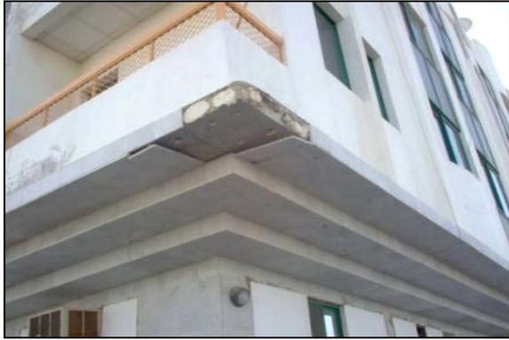
Figure 8. Falling of External Marble Cladding
